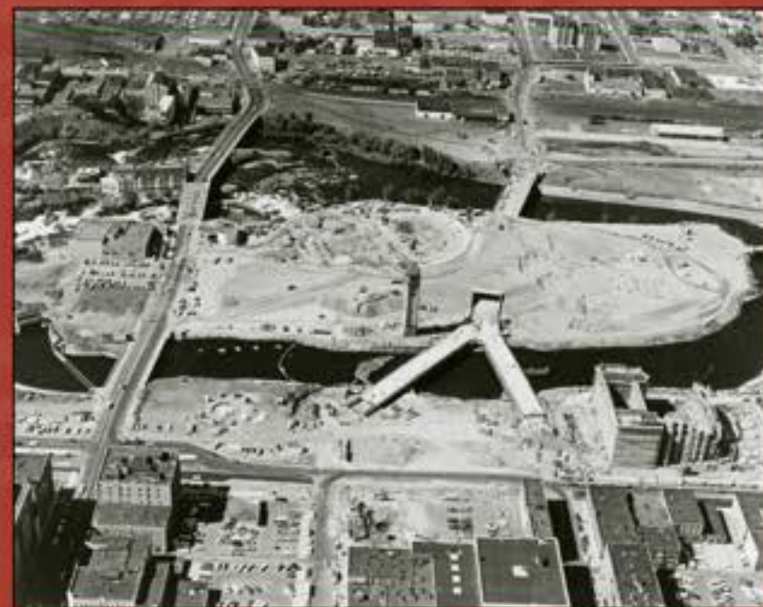
This aerial from 1972 shows the demolition of buildings on the corner of Trent Avenue and Stephens, which housed the last remnant of Trent Alley. From General Photograph Collection, EWU Archives and Special Collections
